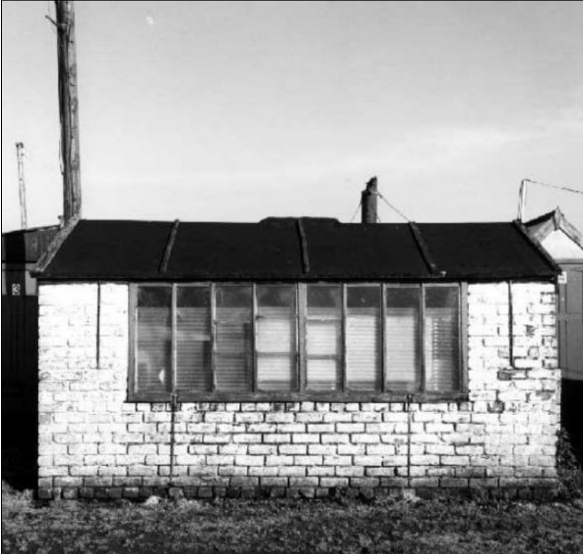
Plate 4 View of a building within Ashton Moss © Tameside MBC
